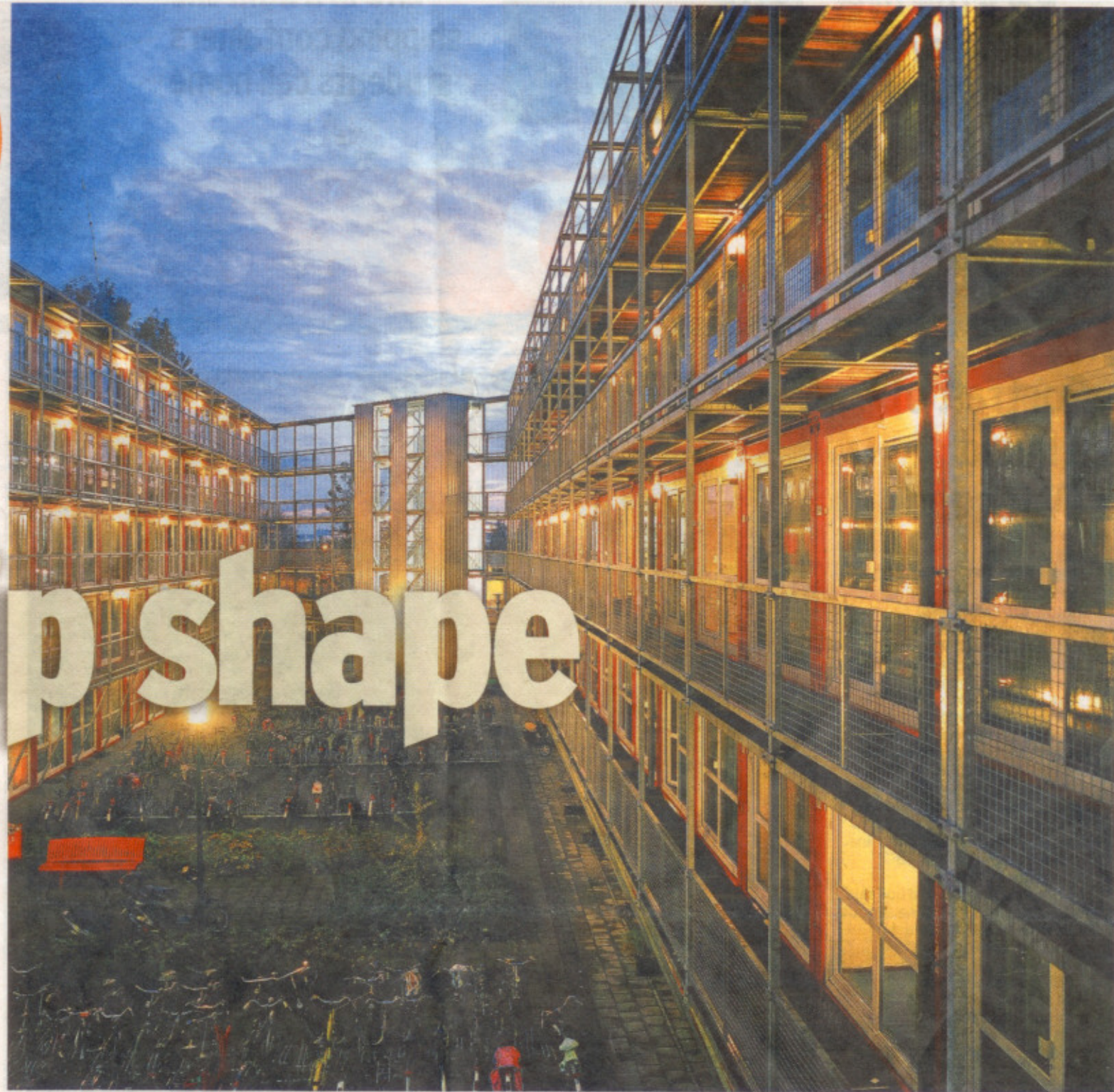
Cheap living ... stacks of containers have been converted into affordable student digs in Amsterdam.
