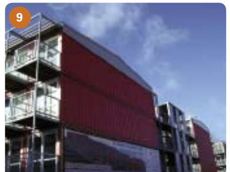
Additional roof for increased insulation and rainwater handling;
