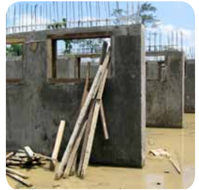
basement under construction
