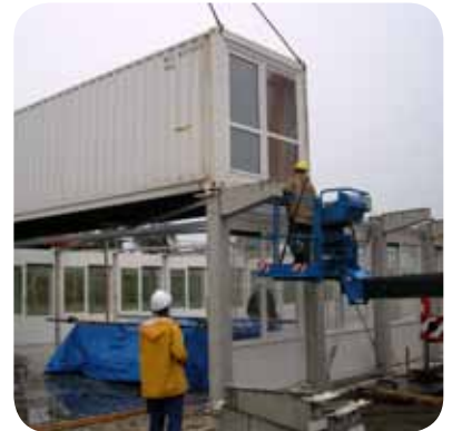
stacking unit on concrete columns
