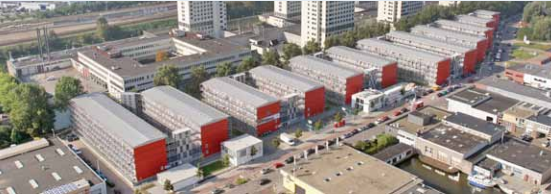
bird's view of the container village
