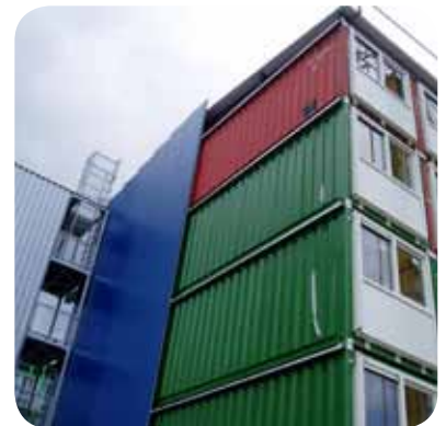
cladding on used containers
