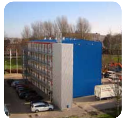
staircase as stability construction
