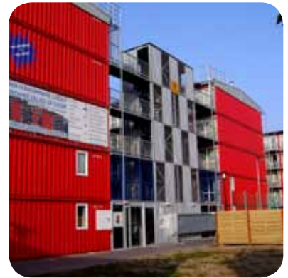
enclosed building block
